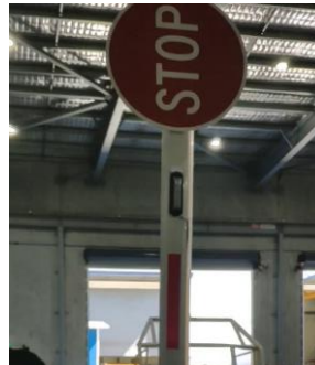
Ensure the orientation of the arm is such that the STOP sign faces the incoming motorists
